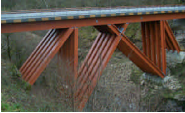
Figure 5.1a – Pont de Merle
