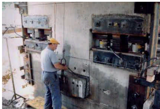
Figure 6.2 – Installation de la pile Koppigen
